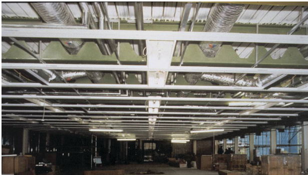
Fig. 2-5. Openings utilized for conduit and HVAC routing.
