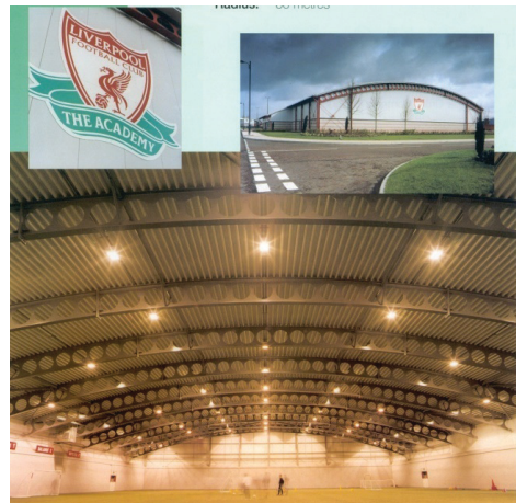
Fig. 2-8. Curved cellular beam roof structure.
