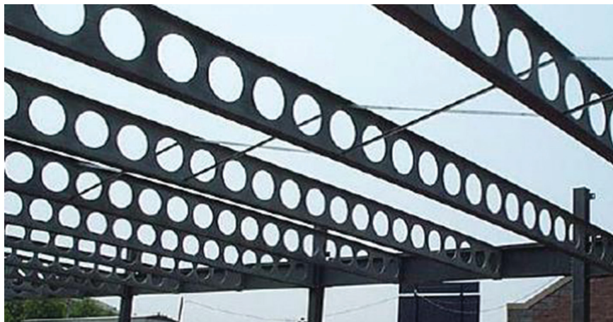
Fig. 2-13. Typical erection bracing for cellular beams (similar bracing used for castellated beams).
