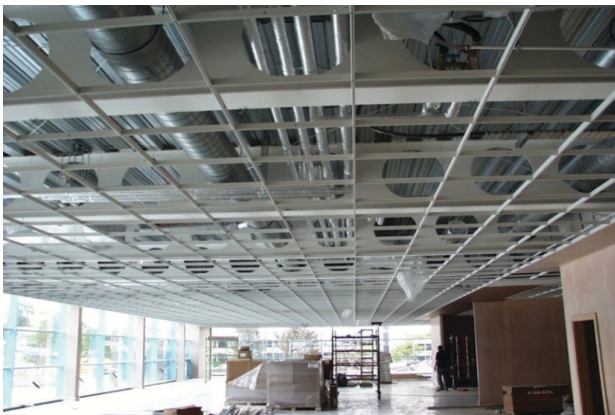
Fig. 2-6. Service integration with ceiling attached to structure.
